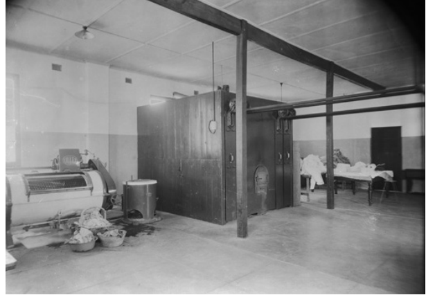
Facilities at Castledare, laundry, 1950. Photograph from Dease Studios collection. Source: State Library of Western Australia .
