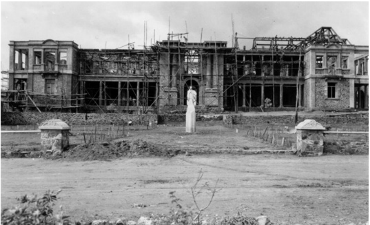
Bindoon Boys’ Town, building work, 1952. Photograph from Western Australia Government photographer. Source: State Library of Western Australia .
