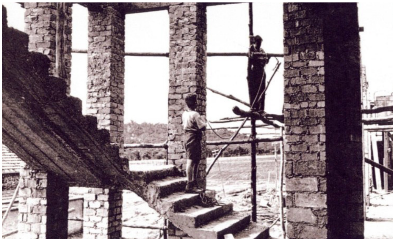
Bindoon Boys' Town, building construction, 1952. Photograph from Western Australia Government photographer collection. Source: State Library of Western Australia .
